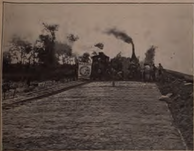
7-Mile Concrete Road, Cedar Point, Ohio
